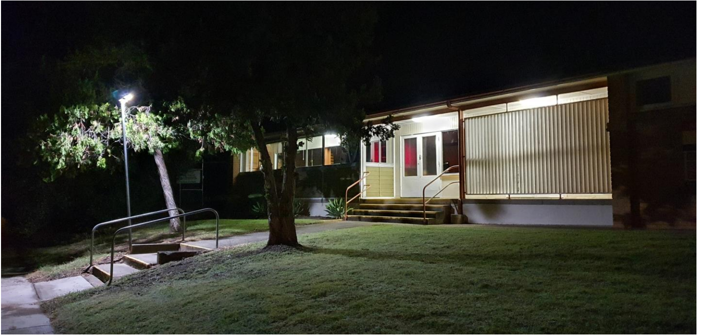
View from Church Street: floodlight over footpath stairs replaced as well as middle light on verandah.
