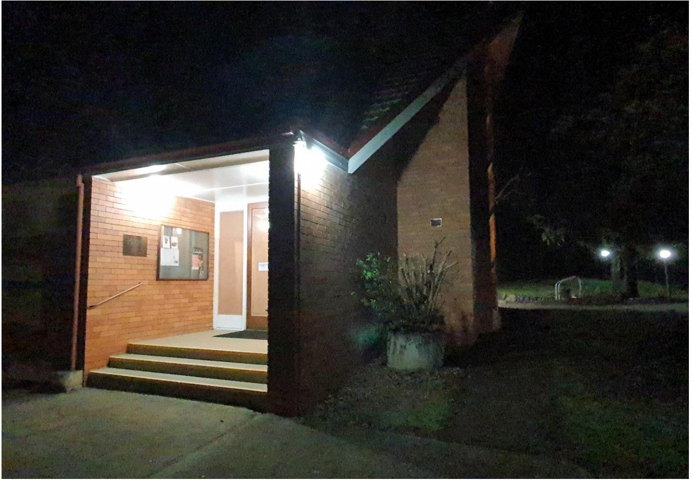
Entrance lights replaced and the corner light on church side reinstalled.
