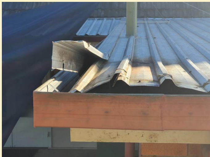
(above) roof damage from where the bracket holding the sail was ripped out by the wind; (right) damaged sail over the concrete gathering area at the side of the Boonah church.
