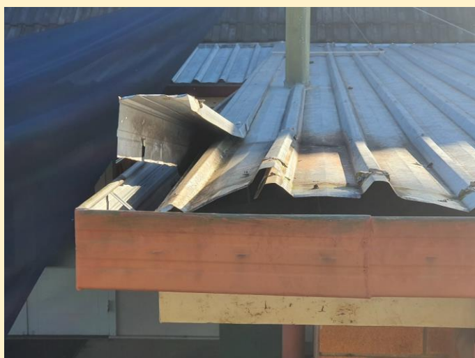
(above) roof damage from where the bracket holding the sail was ripped out by the wind; (right) damage sail over the concrete gathering area at the side of the Boonah church.
